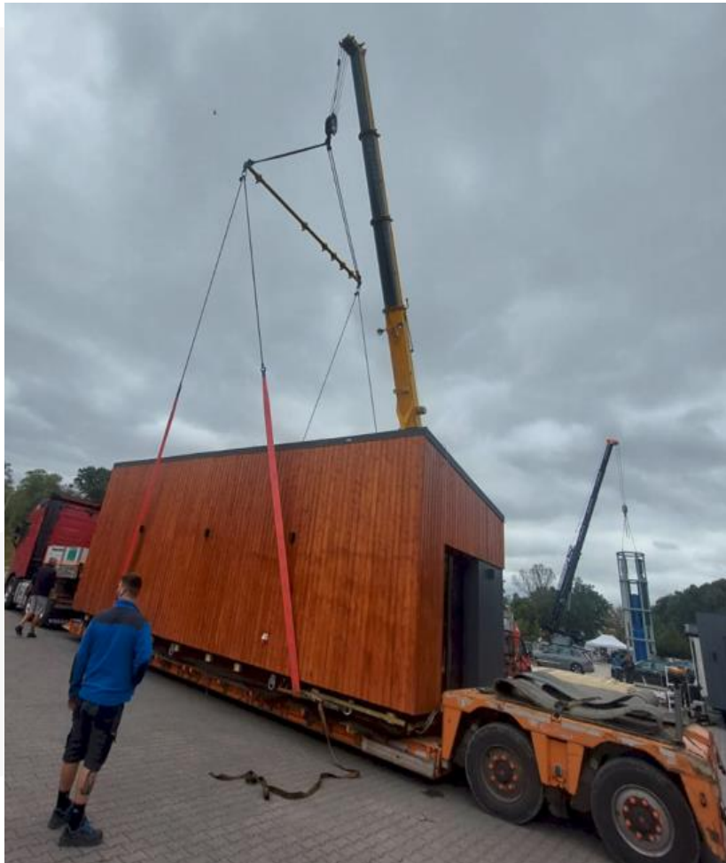
Fig. Example of unloading using a spreader bar.
