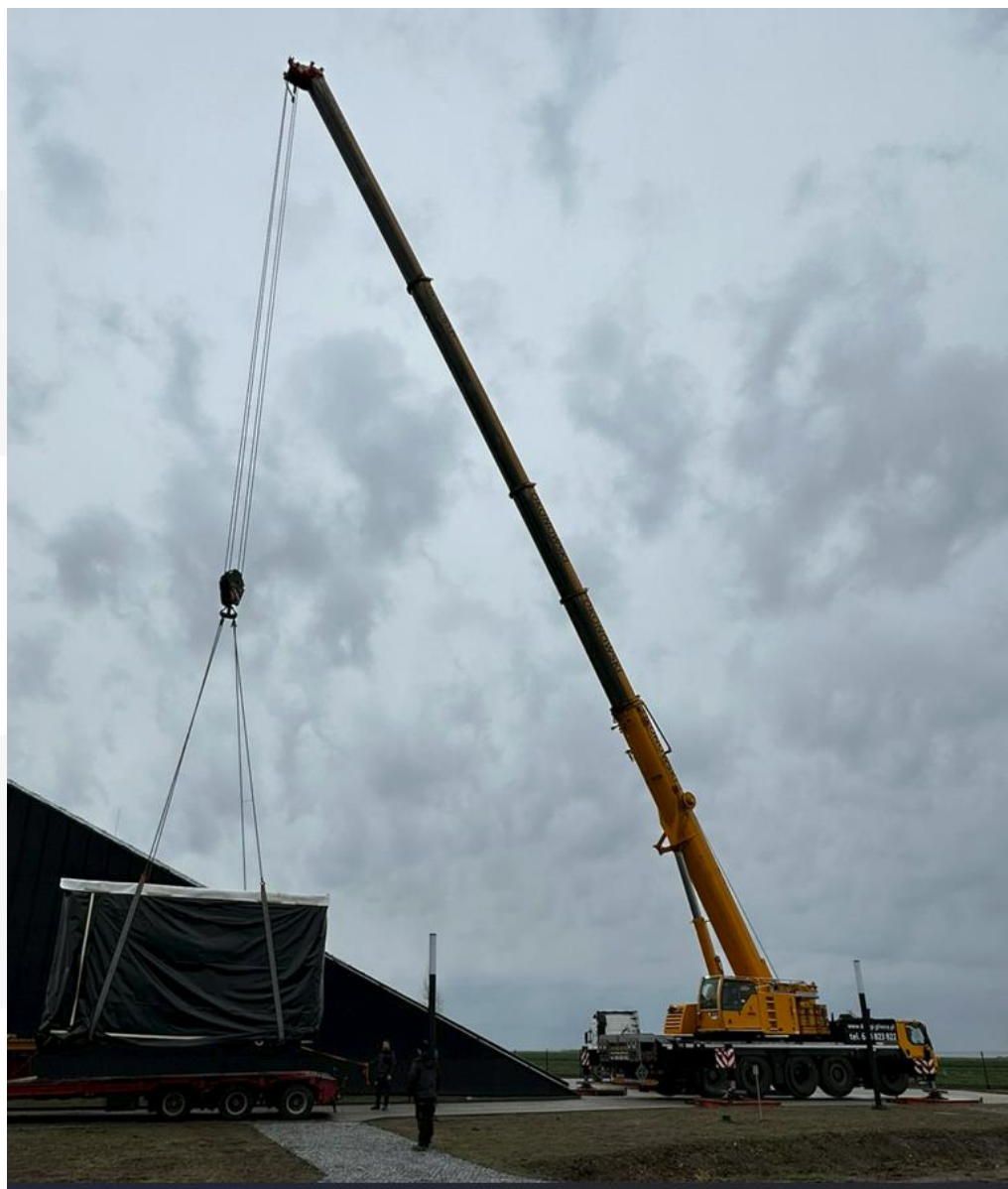
Pic. Example of unloading without using a spreader bar.
