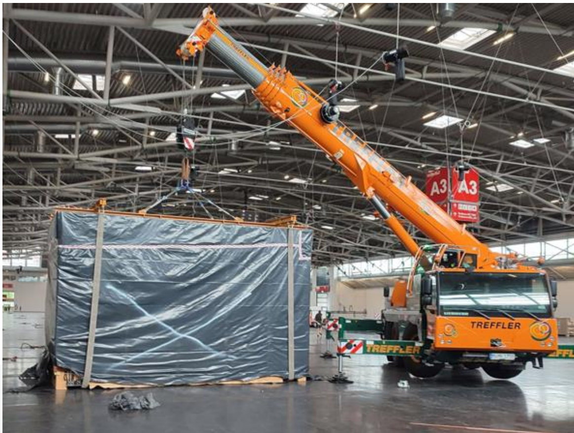
Fig. Example of unloading using a H-type spreader bar.
